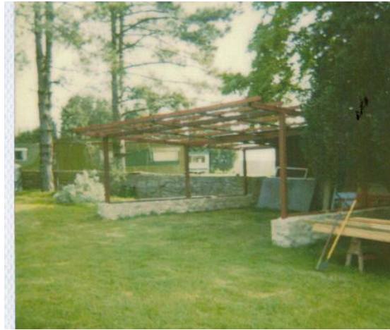
Carport building in 1992.
