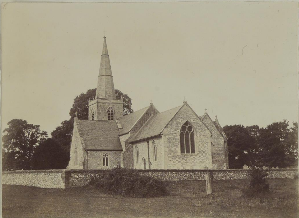
Martin Church after Restoration in 1897
